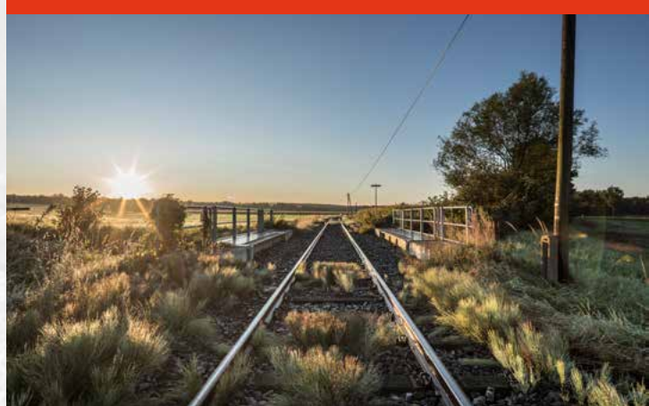
Photo: Open Rail Lab
